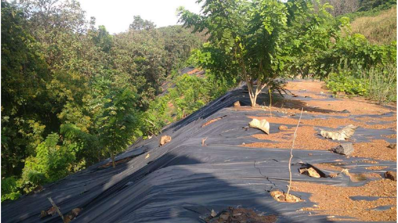
Photographs showing the top soil and OB storage area
